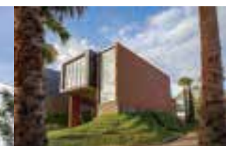
THE VICTORY BY ANDAMAN ASSET SOLUTION
